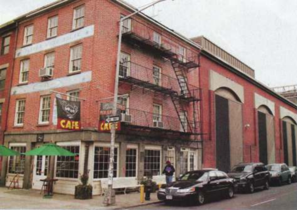
RADIATION THERAPY: Aluminum panels separate Polumbo's home (above café) from Con Edison.
